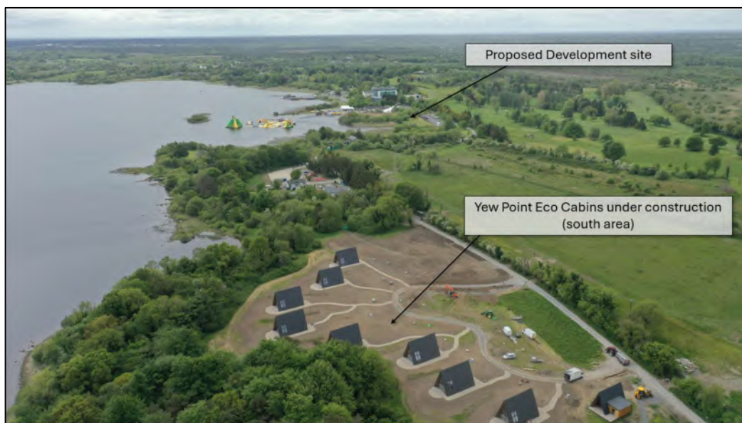
Figure 13-21 Drone imagery looking south, of Yew Point areas currently under construction (as of May 2026) for the eco cabins development and position relevant to the Proposed Development Site
