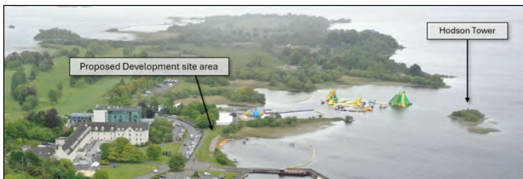
Figure 13-17 Drone imagery facing north, showing the overhead landscape view of Hodson Tower location relative to the Site
