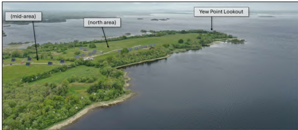
Figure 13-23 Drone imagery facing northwest, of mid-area and north area of Yew Point Eco Cabins under construction and position relevant to Yew Point Lookout
